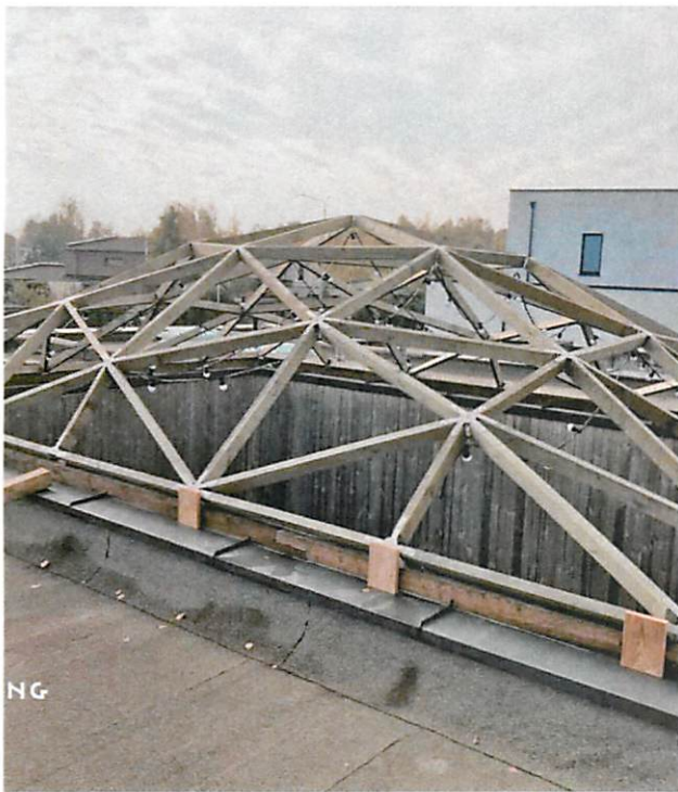
8x9m Quadro dome rooftop cover in Vilnius, Lithuania
